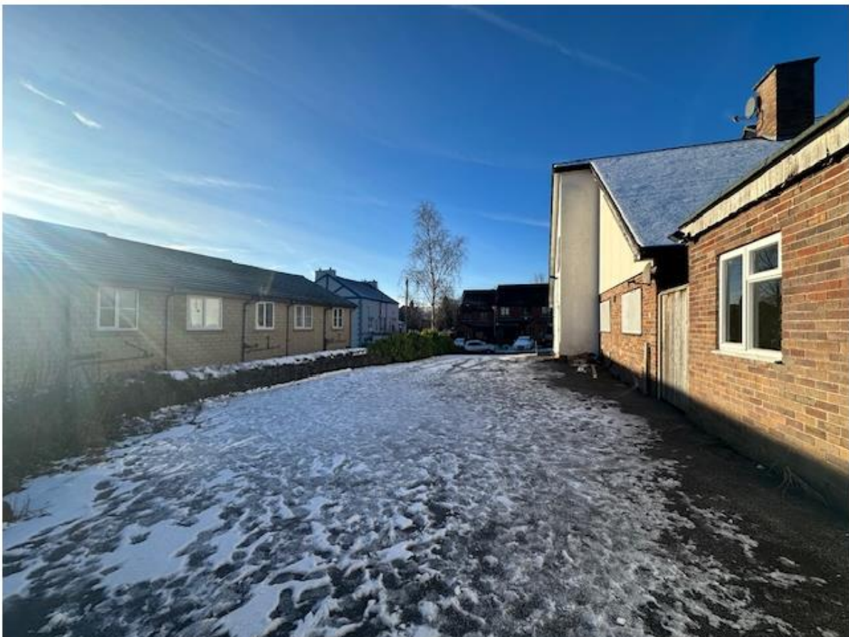
Image 4: view of Spring Court Mews from existing hardstanding area to south of plot
